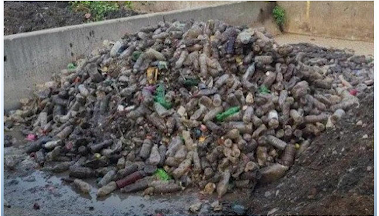
ONE DAY OF CLEANING PROVIDENCE PLACE MALL SIPHON INLET STRUCTURE
