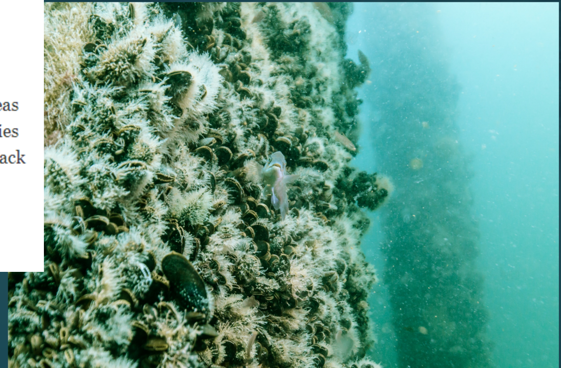
Sea life on the Block Island Wind Farm foundations
