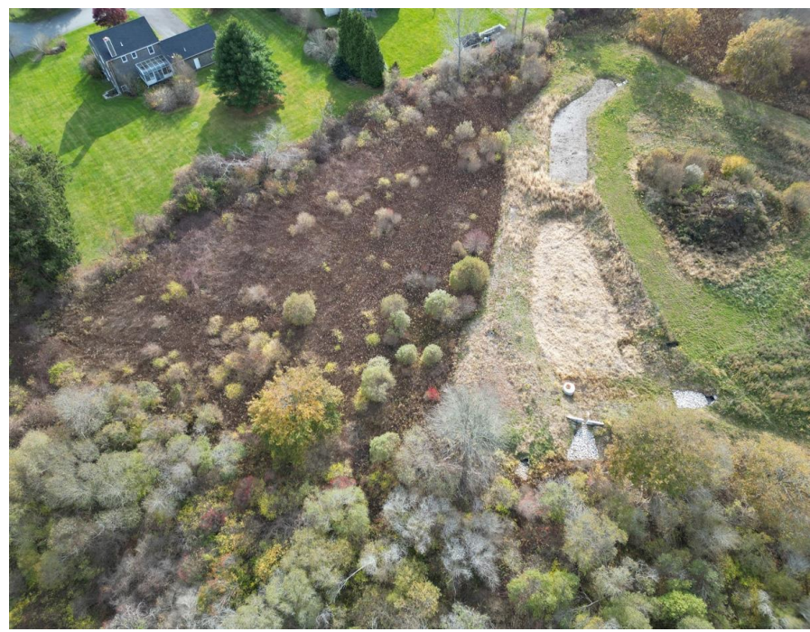
Drone photo taken from the north, looking southward at encroachment area on November 12, 2025.
